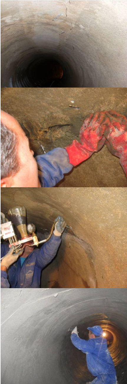
Picture 3. Phases of executing of the work in derivation channel
