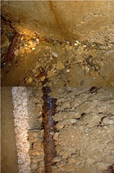
Picture 2. Conditions of the structure during the evaluation moment
