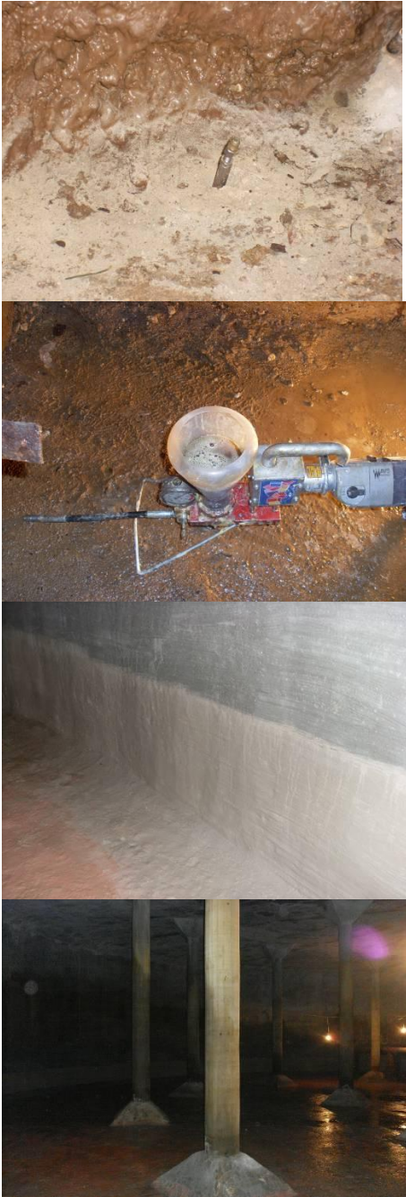
Picture 5. Repairing steps in the water tank
