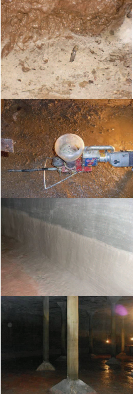
Picture 5. Repairing steps in the water tank
