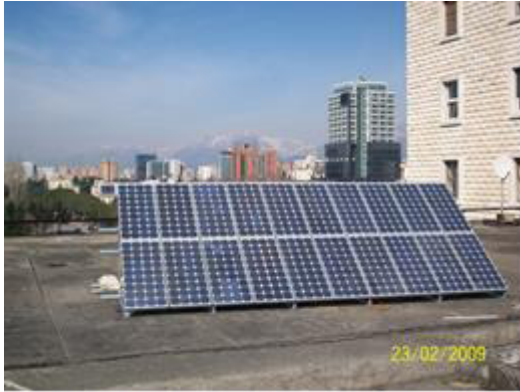
Figure 1. 1500Wp Photovoltaic Panel
