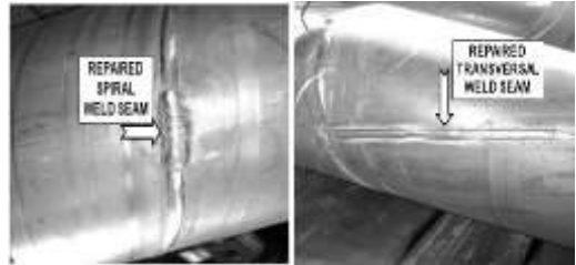
Fig.4. Visual control of the repaired weld seam
