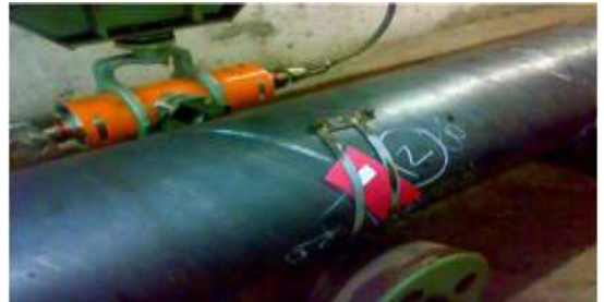
Fig.5. X-ray control of the repaired weld seam
