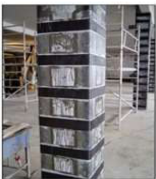
Figure 2. Applications of FRP reinforcement in columns [10]
